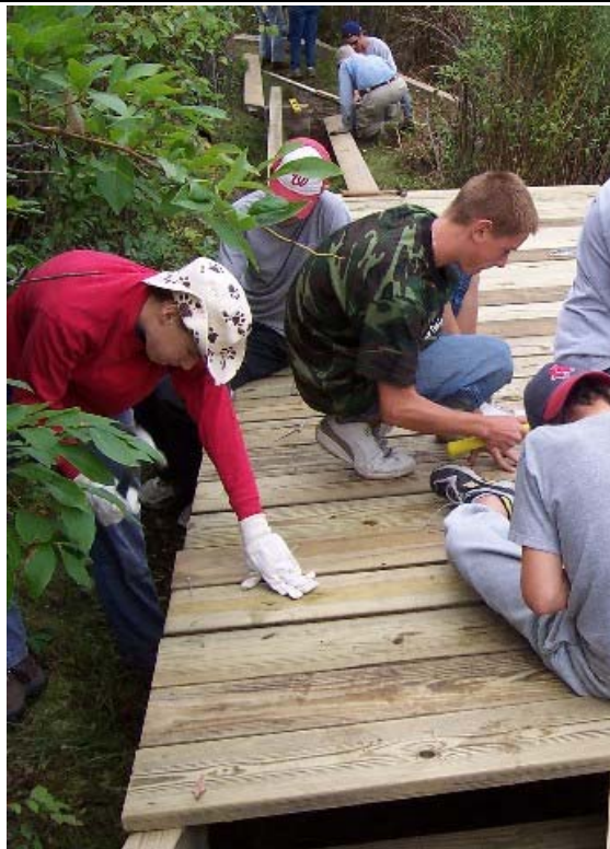
September Boardwalk Work
