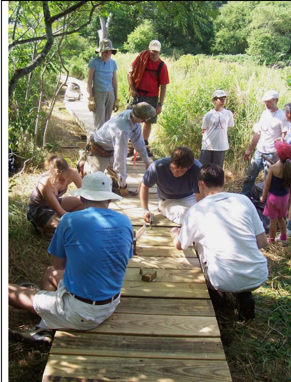
July Boardwalk Construction
